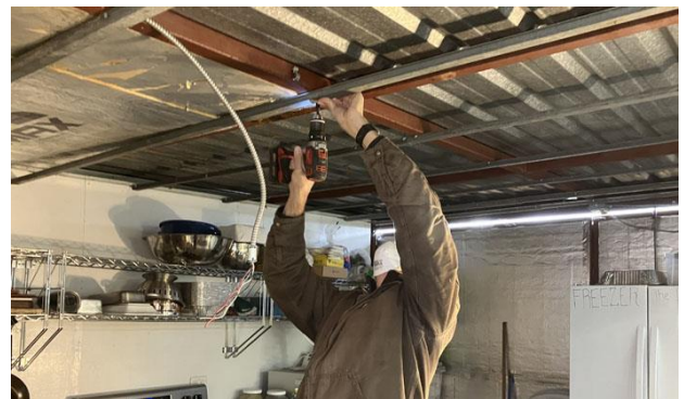
Insulation going in. Cool in summer, warm in winter. Comfy cooking in the clubhouse kitchen.
