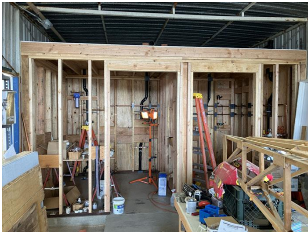
We've been framed (and plumbed...)
